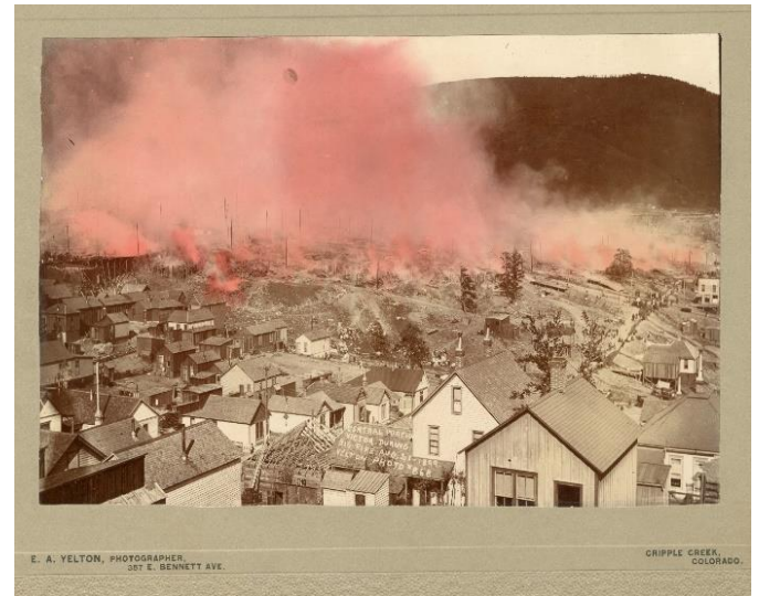
Figure 6 The fury of the Victor fire on August 21, 1899, photographed by E. A. Yelton. Photo courtesy of the Cripple Creek District Museum.
